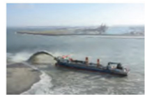
Trailing suction hopper dredger Van Minne working at the Maasvlakte 2 project.
