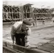
Construction of Velsertunnel (photo Olof Kruger, 1957).
