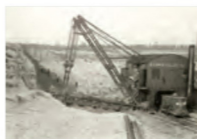
An ABM excavator at the locks in IJmuiden (photo 1926).
