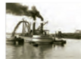
The Humber, a barge unloading dredger belonging to K.L. Kallis (photo L.J. Smit, 1906).
