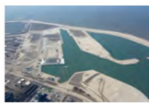
Construction of harbours in Rotterdam remains important for several major dredging companies right into the 21st century. This photo shows Maasvlakte 2 (photo 2013).
