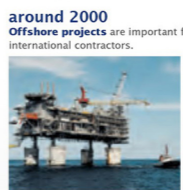
Malaysian offshore installation project, the Philippines.
